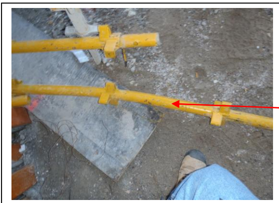
Bent scaffold standards as a result of overloading
