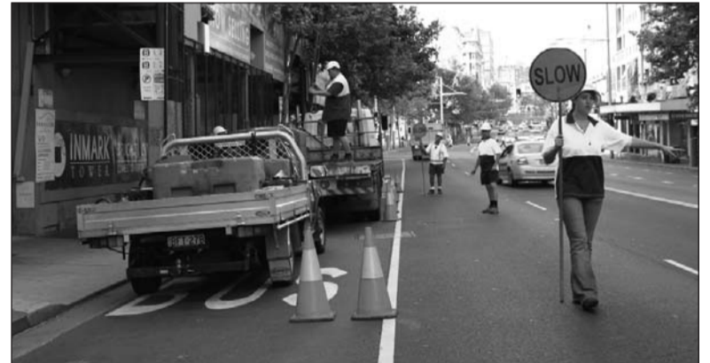
Three traffic controllers are now employed and new safety procedures for unloading/loading trucks by crane are in place.
